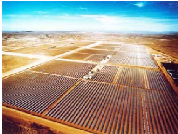
Aerial photo of the SEGS plants in Kramer Junction, California.
