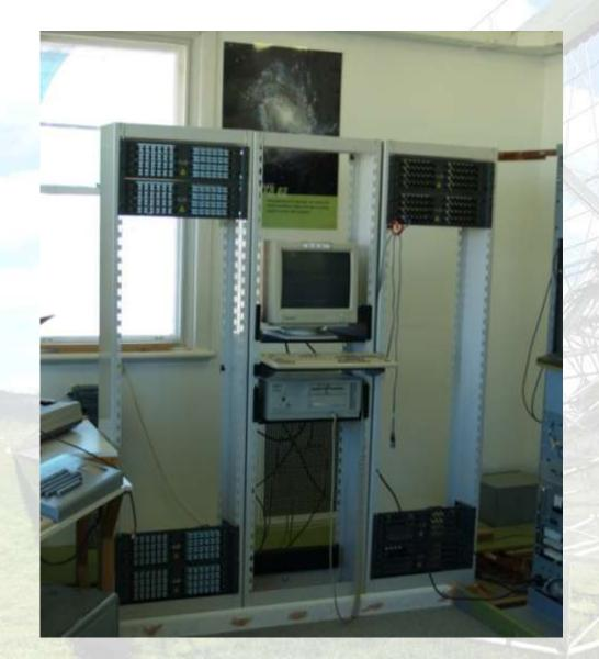
Racks installed for fibre patch panels, polyphase filterbanks & correlator.
